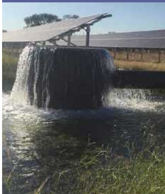
FIGURE 3: An industry first installation of a 55 kw submersible pump driven by combined 100KW solar and 110 kVA diesel generator at the Gill family's 'Waterloo' Narromine, NSW. (Photo: Jon Welsh)
