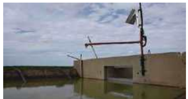
Monitoring and maintaining consistent channel head heights ensures more even siphon flow rates and more efficient irrigation. (Photo: Lou Gall, GVIA)
