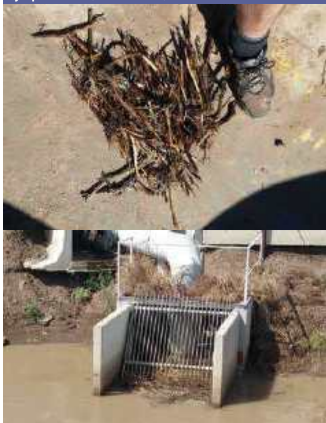
FIGURE 2: Cotton trash can reduce pump performance by up to 30%. (Photo: Phil Szabo)
